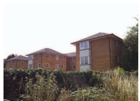
adjacent properties to the South
