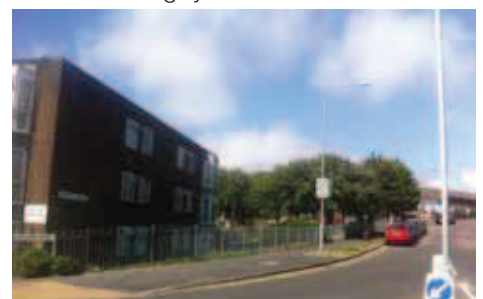
view from Whitehawk Road along Manor Way
